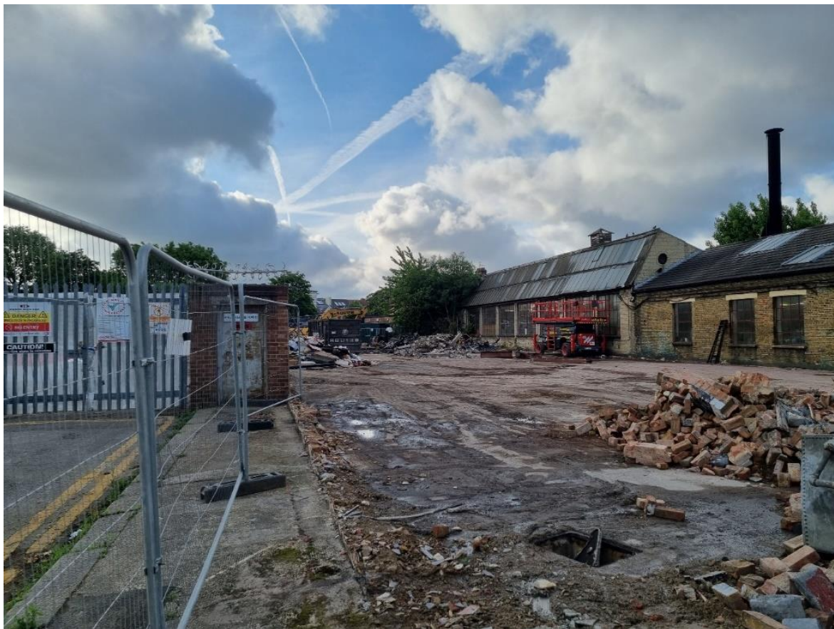
Work underway clearing site at Ashley Road, Tottenham Hale
